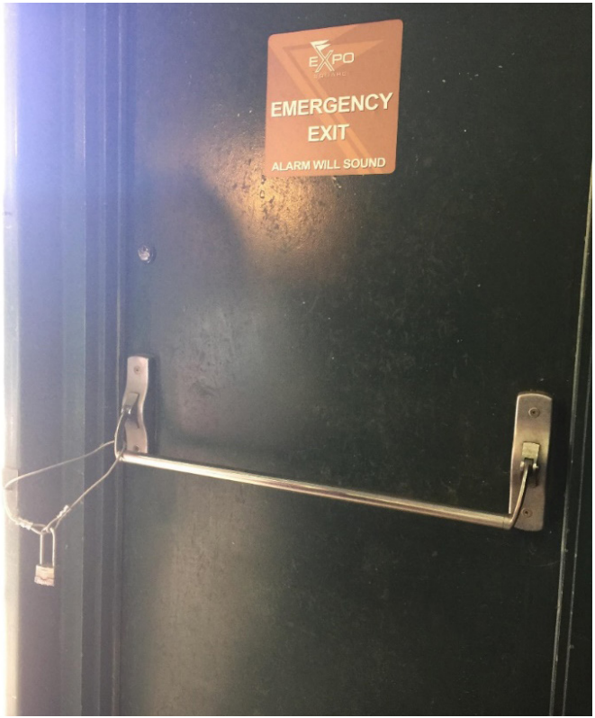
Egress door with push bar and pad lock
