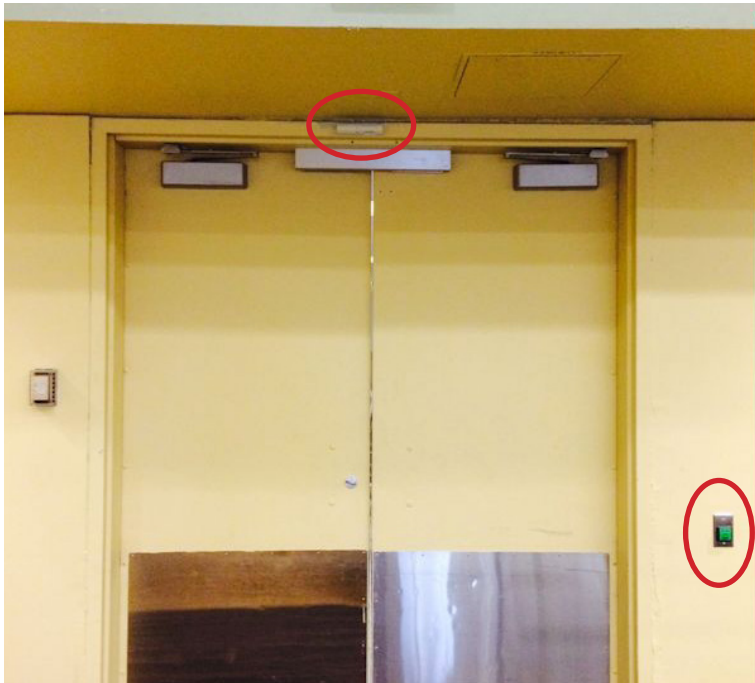
Motion sensor and push to exit button provided on egress side of door with electromagnetic locking device
